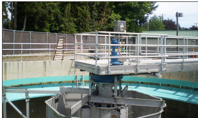
*The WWTP's secondary clarifier, previously performing dual process functions of secondary clarification and WAS thickening, was rebuilt and set back to its intended purpose of providing additional plant capacity.*
